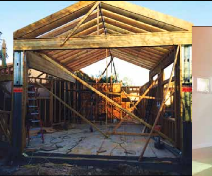
Framing of the studio roof
